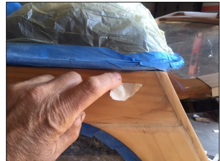
Repaired water stained wood
