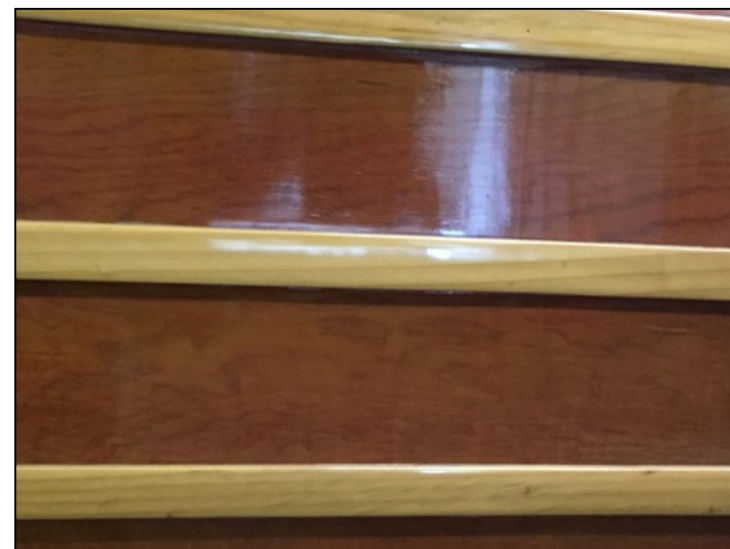
Finished wood on doors
