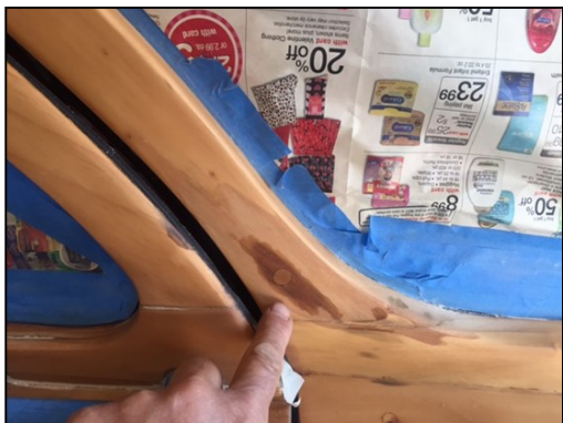
Water stain removal in process
