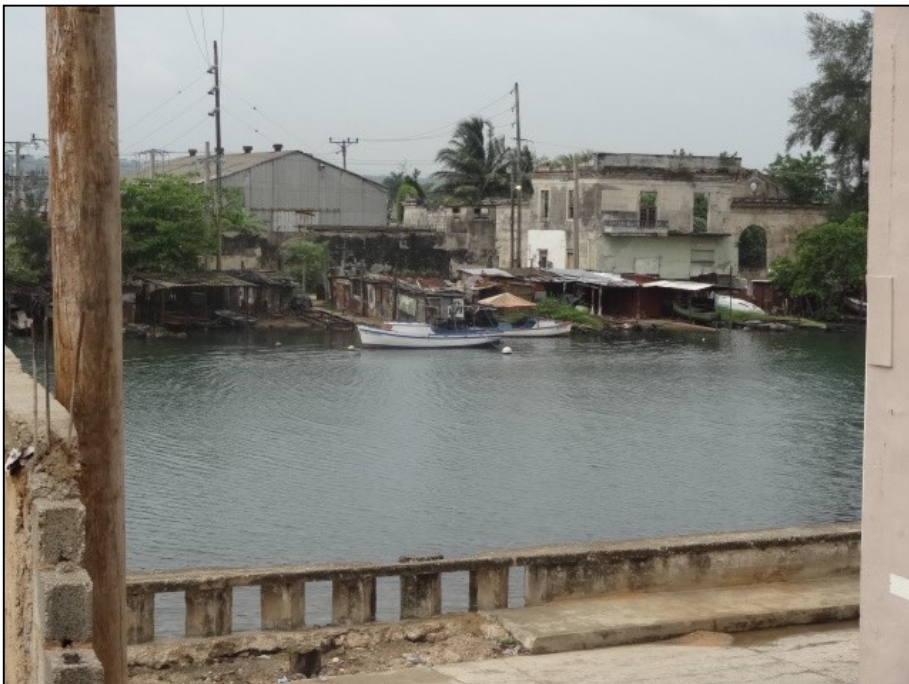
Poor conditions in Cuba. Notice the decaying concrete in the foreground.
